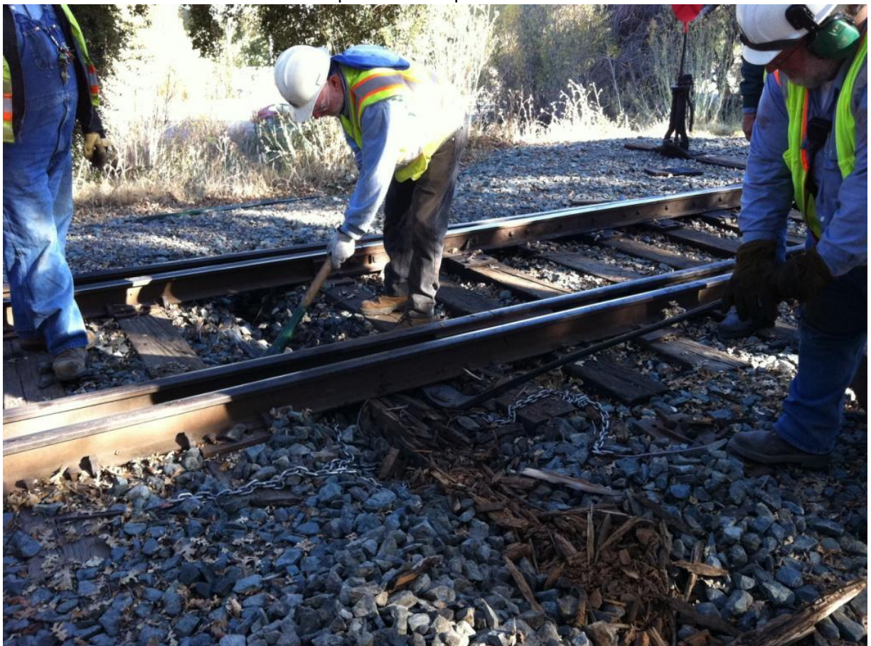
The tie disintegrated into splinters. The only solution is to dig it out by hand.
