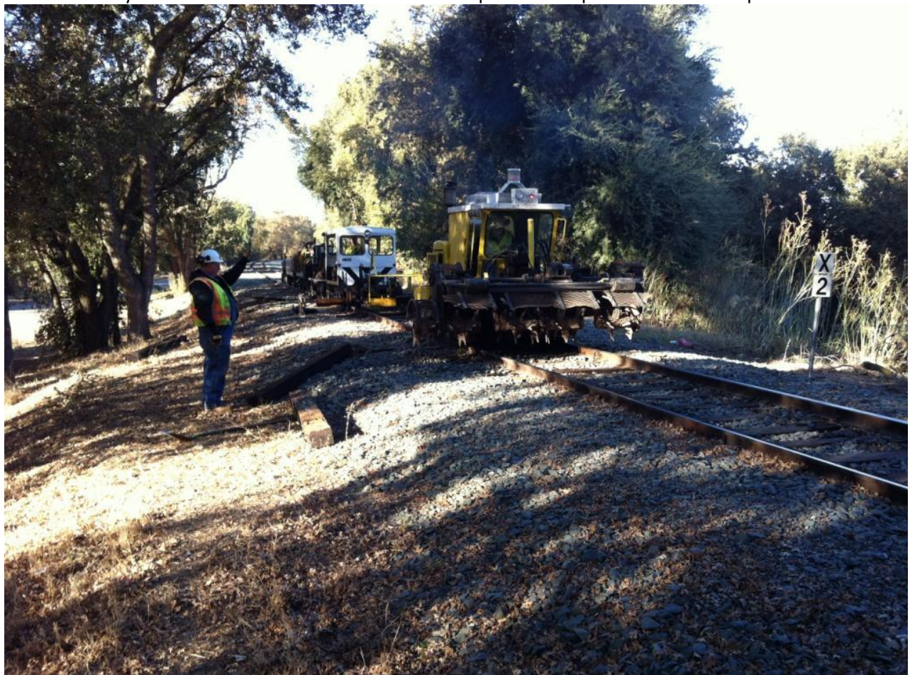
Chris guides Alan in the scarifer to line up with the now empty crib of the removed tie
