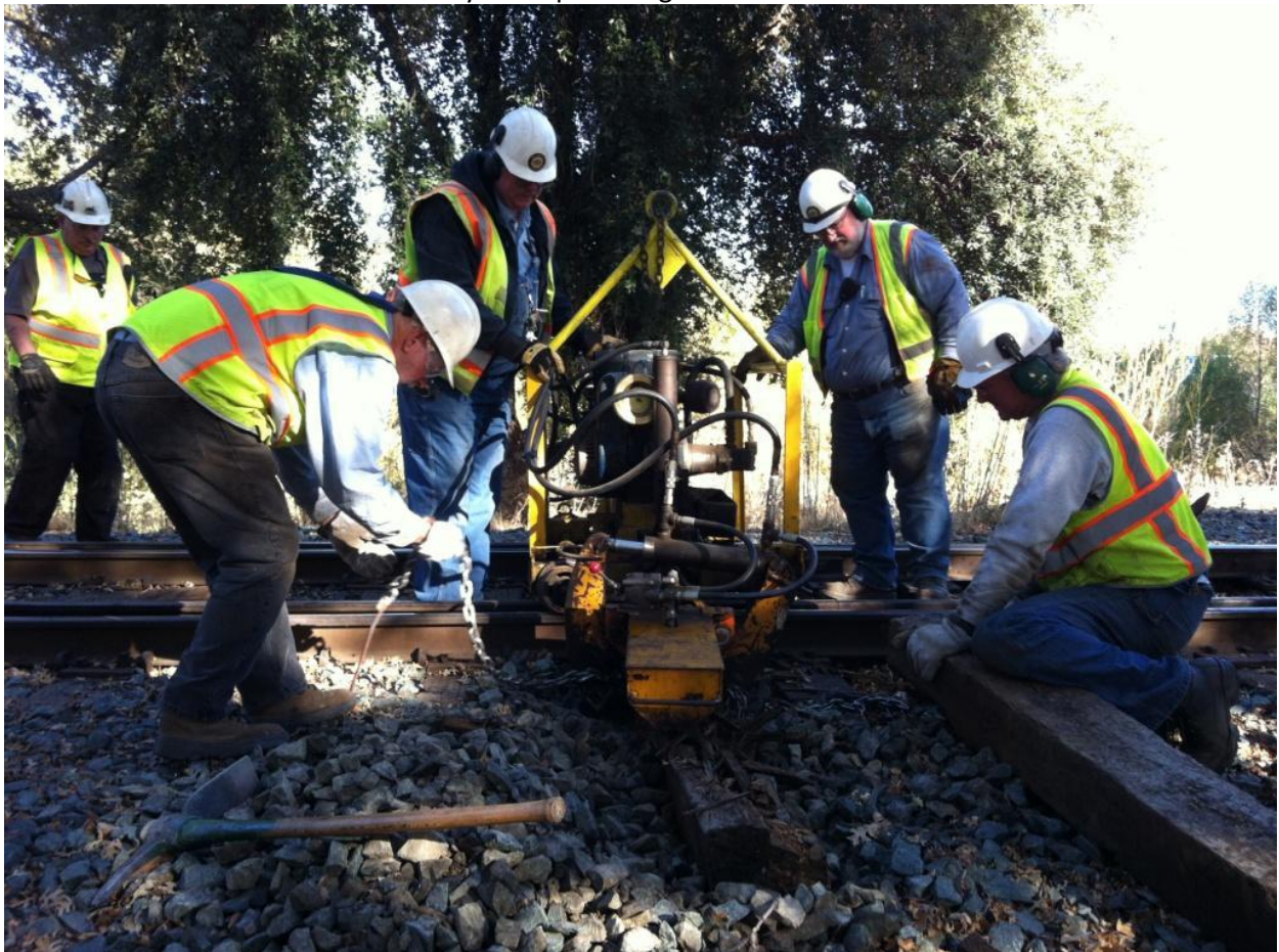
Mike, Chris, Frank, and Steve use a chain to pull the rotten tie out with the section-gang machine
