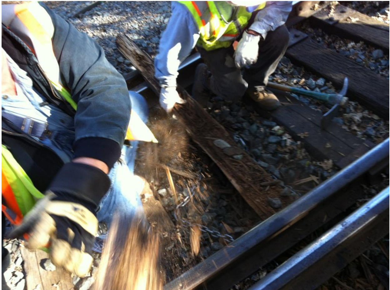
Action shot: the tie “explodes” into splinters as we work to remove it
