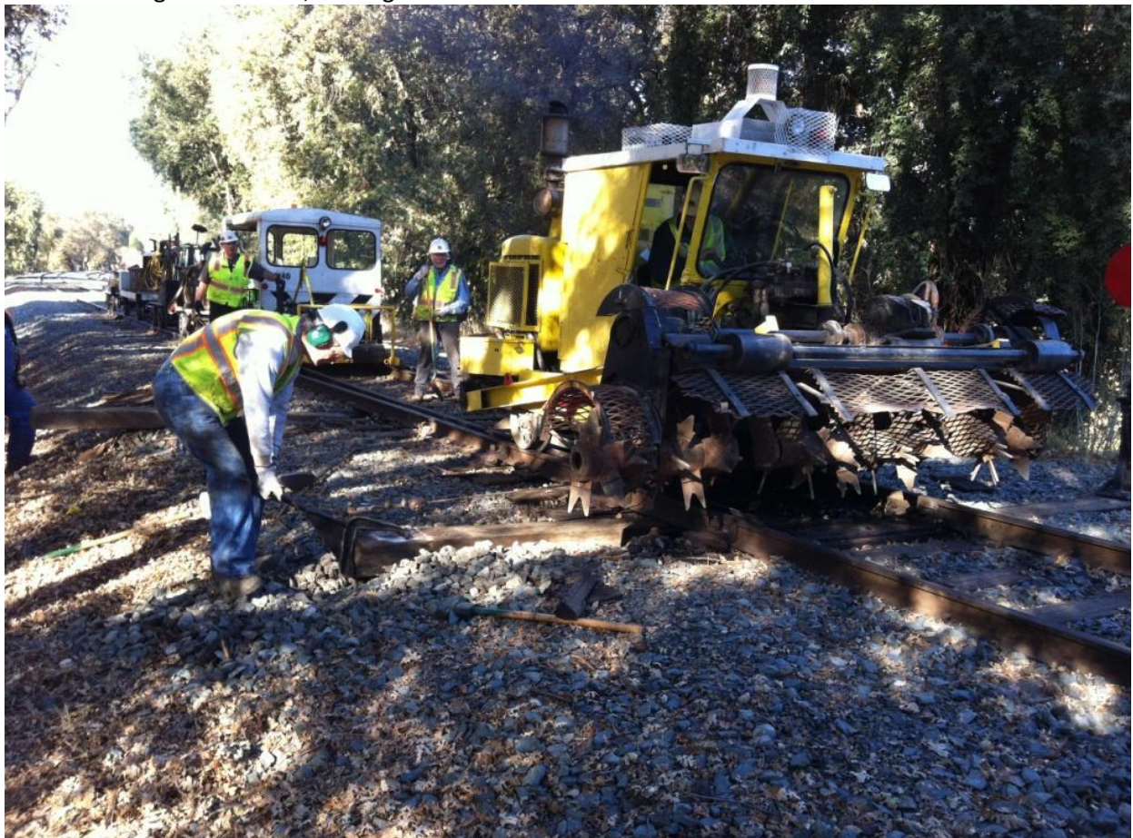
The new tie being pulled into place
