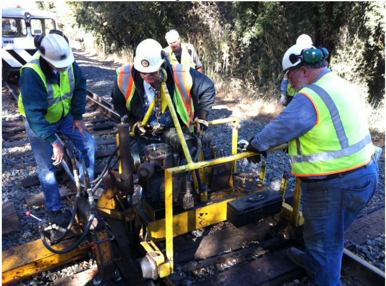
Alan, Chris, and Frank work with the section-gang machine as it crushes the rotten tie they're trying to pull...
