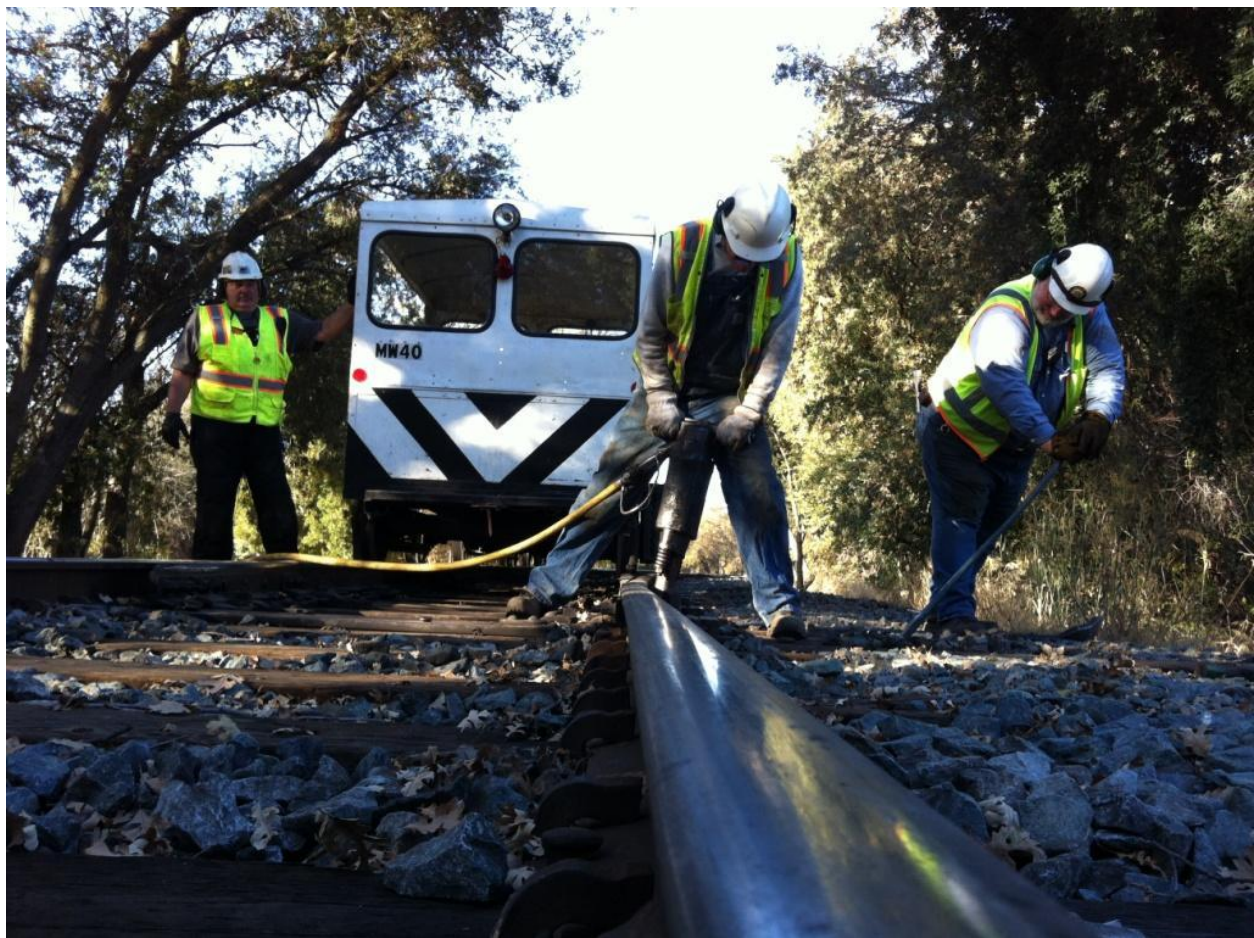
Harry at the helm of the A-4 as Steve uses the pneumatic spiker while Frank nips the tie
