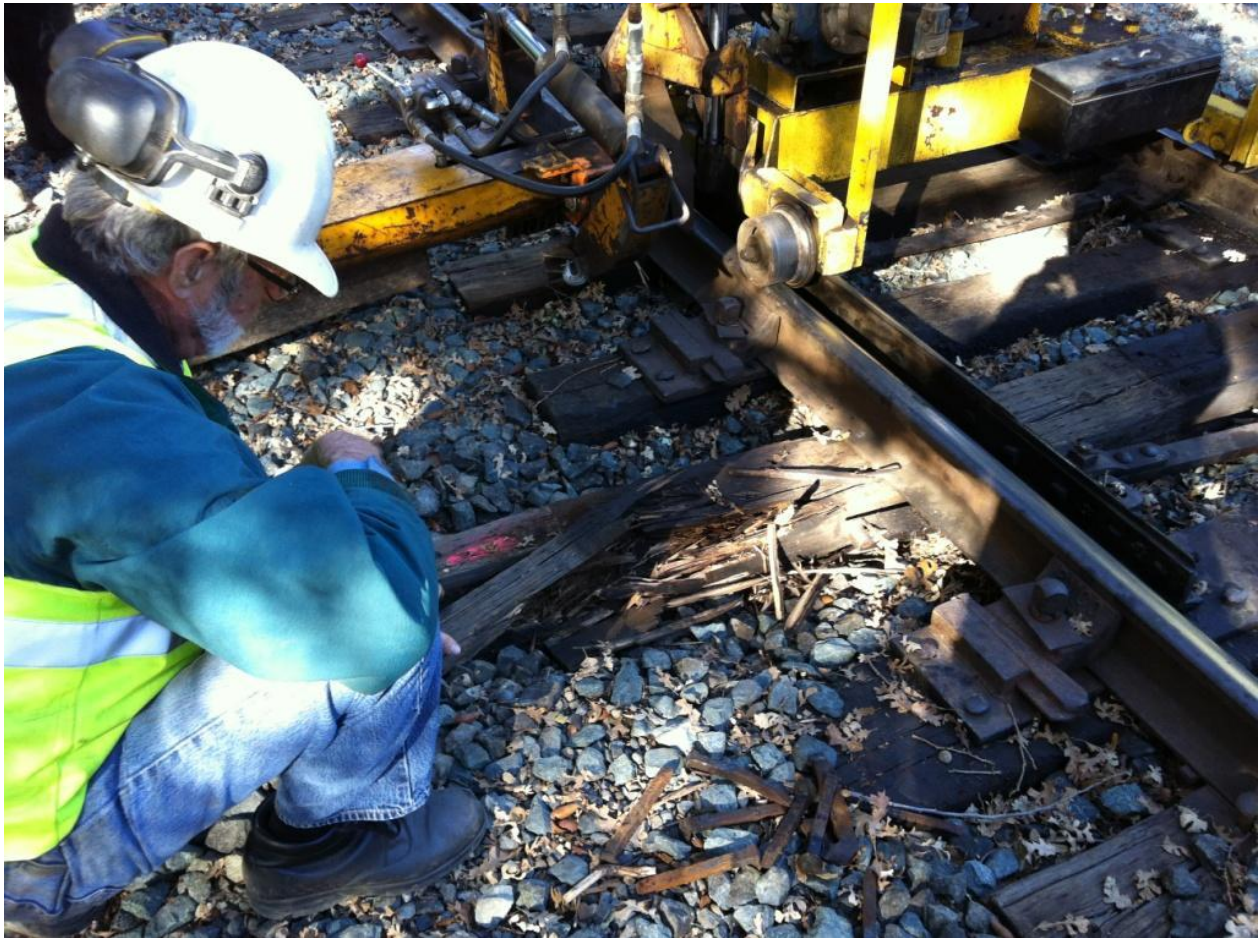
Alan surveys the splintering tie beneath Switch 16
