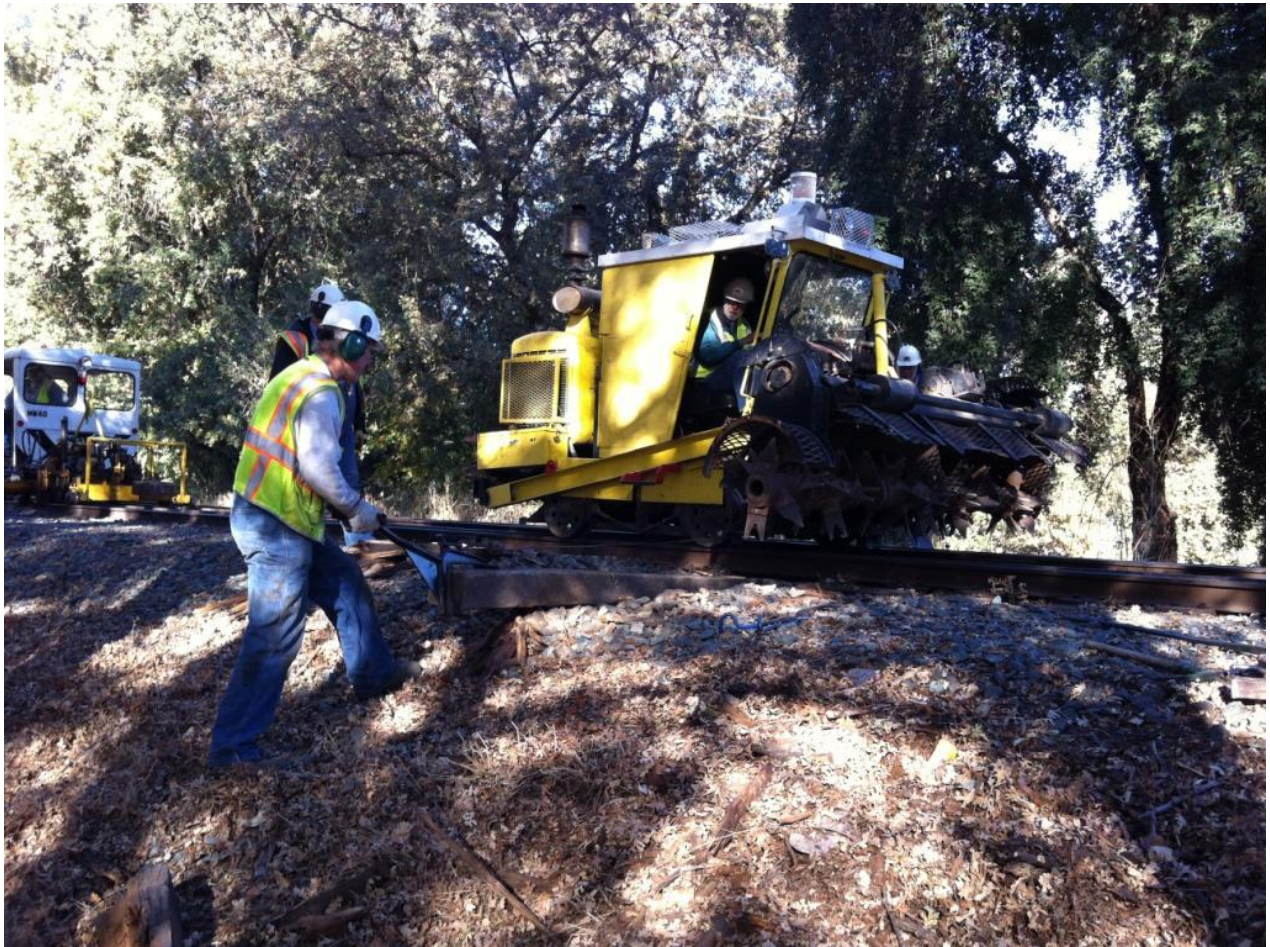
With the offending tie removed, Steve guides the insertion of a new hard-wood oak tie with Alan on the Scarifer
